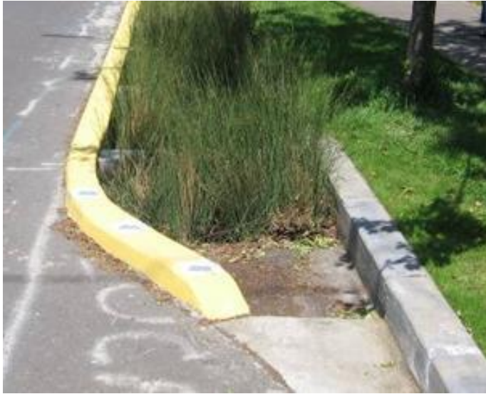
Figure 14: Example of a stormwater curb extension for the Route 7 ROW (Credit- VA DRC Stormwater Design Manual 2013).
