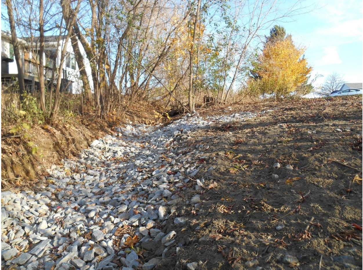
Figure 8: New stone cover in existing drainage swale, near location of proposed infiltration basin.
